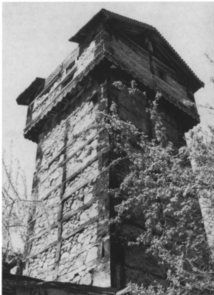
Fig. 3: Fortified tower in Harban-kot, belonging to the Miańkulé lineage
